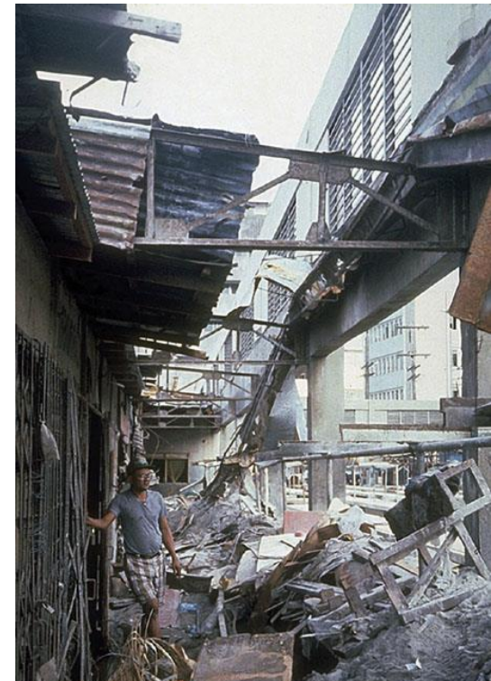
Ashfall from Mt. Pinatubo collapsed many roofs
