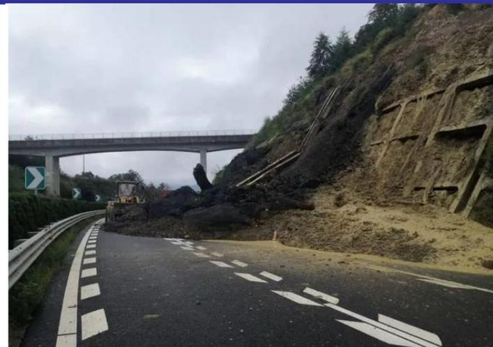
$$FOS = \frac{T'_R}{T_R} = \frac{T'_R R}{T_R R} = \frac{\sum cL_i + (W_i \cos \alpha_i \tan \phi)}{\sum W_i \sin \alpha_i} \quad W_i = f(\theta, H, \gamma) \quad FOS = f(\theta, H, \gamma, c, \phi)$$
